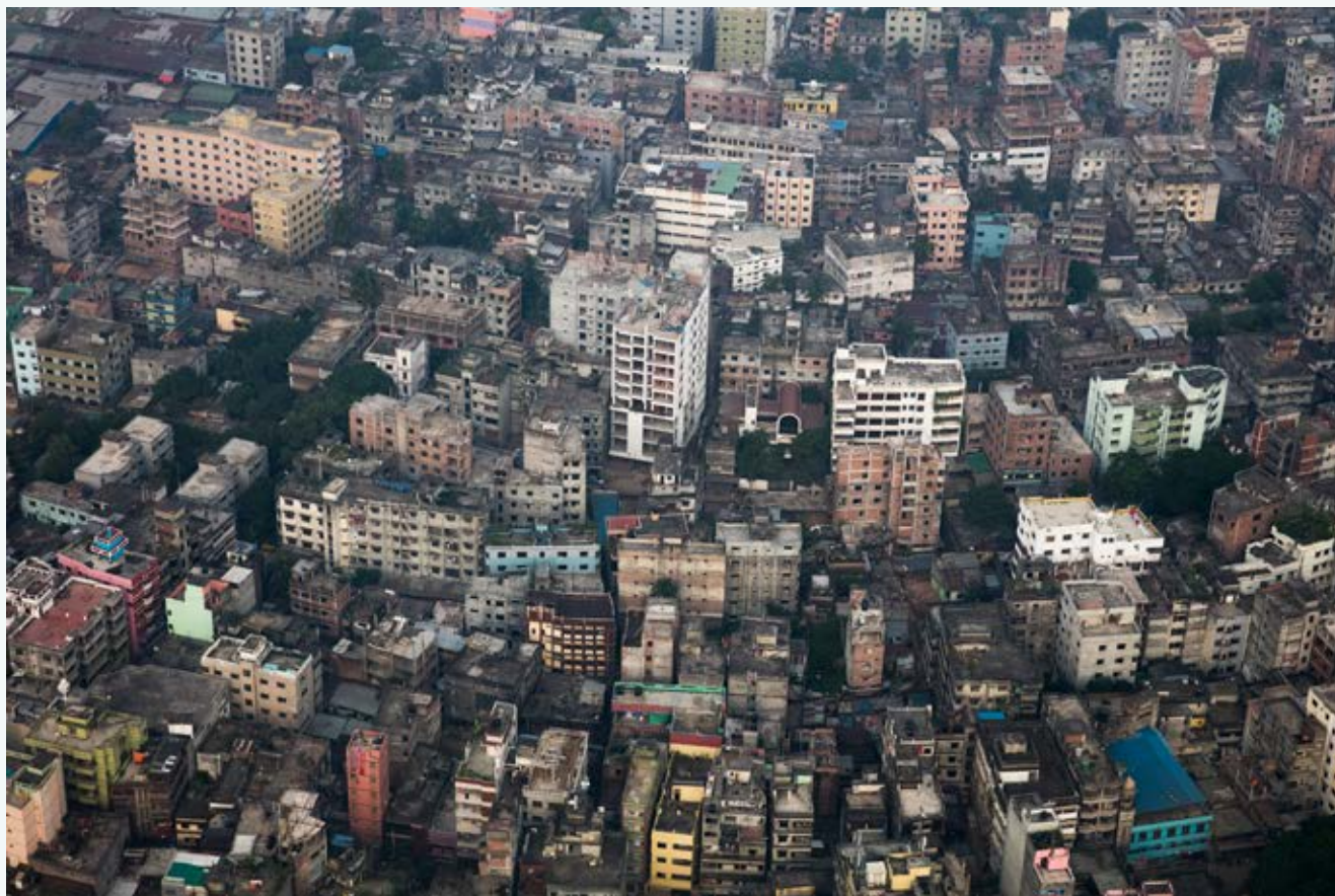
Figure B15.1 | Very high levels of density in the city of Dhaka
