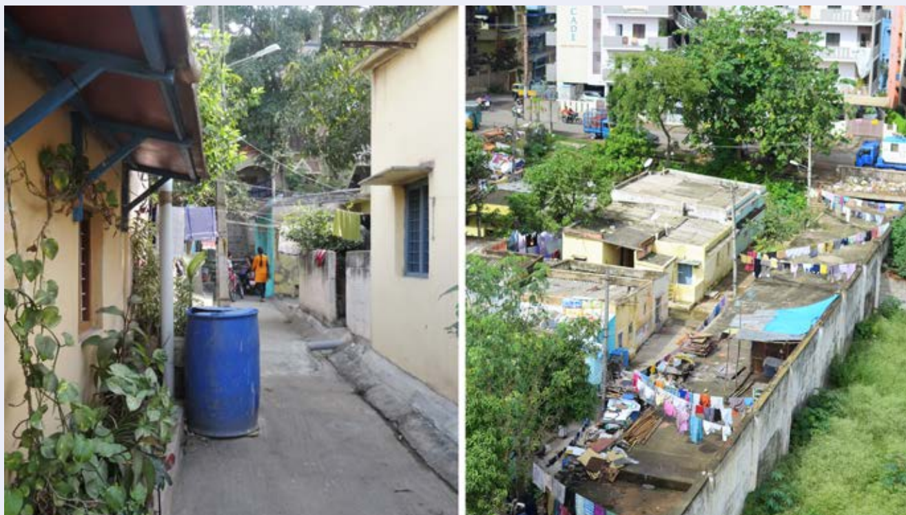
Figure B8.1 | Thulsimma’s neighborhood in Bengaluru suffers from being in a low-lying, flood prone area and piped water is stored in large drums
