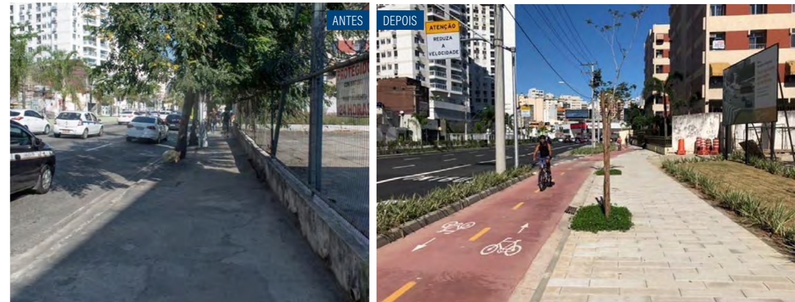
Figure 68 | Before and after the urban qualification: based on a new alignment of the road, it was possible to implement a new bidirectional and segregated bike lane, and to expand and upgrade the sidewalks
