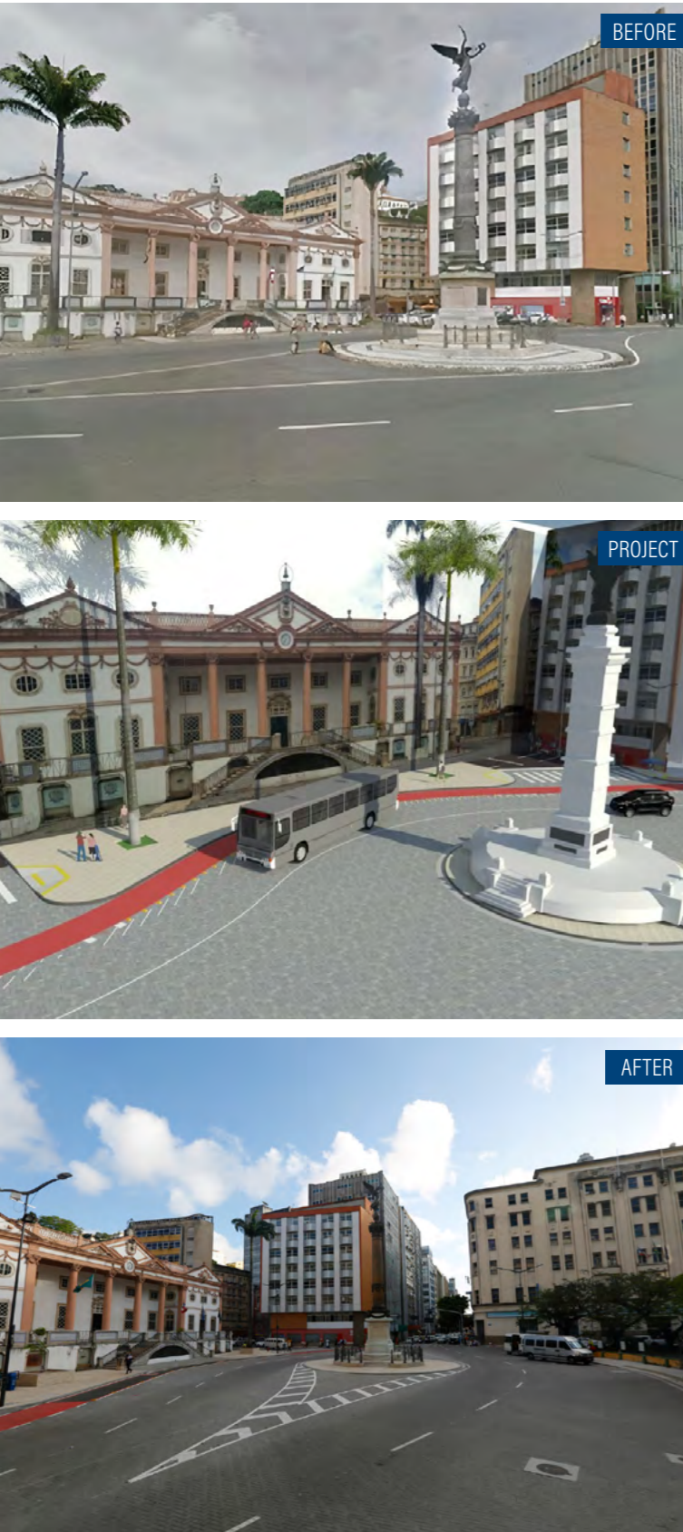
Figure 14 | Praça Riachuelo, before, during the project, and after the intervention
