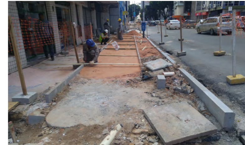
Figura 15 | TSection of Rua Miguel Calmon during the intervention
