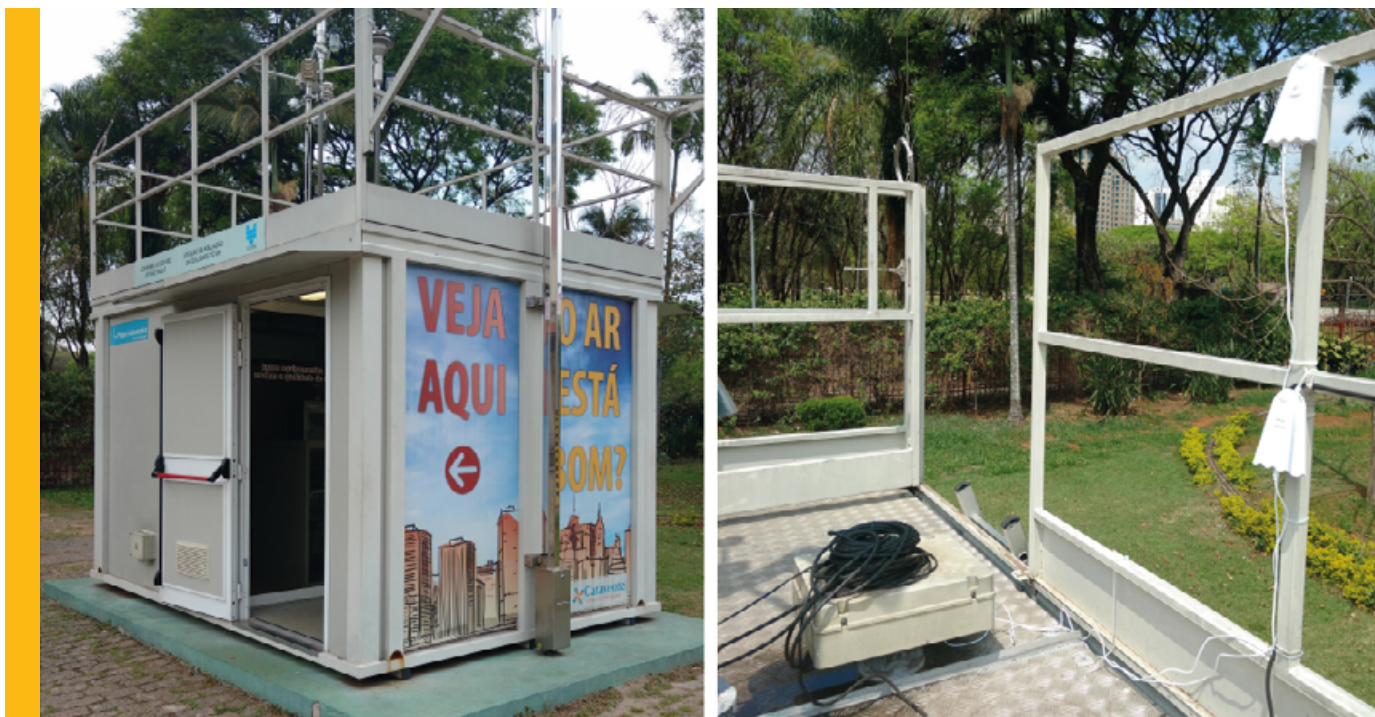
Figure 6 | AirBeams Installed at the Top of the Monitoring Station
